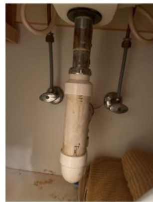
SECOND FLOOR BACK BATHROOM SINK RIGHT SIDE VALVE LEAKS
