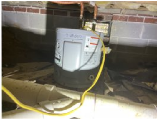
WATER HEATER IN CRAWL
