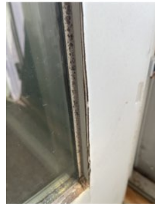
SECOND FLOOR OFFICE DOOR DELAMINATION
