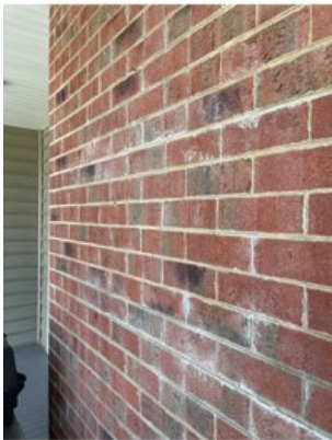
CHIMNEY EFFLORVESENCE
