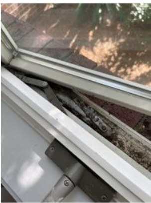
CASEMENT TRACKS AND OPERATOR REQUIRES CLEANING
