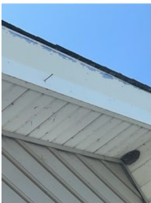
PVC ADHESIVE FAILURE
