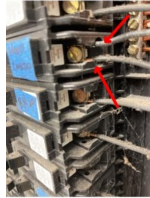
DOUBLE TAP ON BREAKER MARKED HOOD COOK TOP
