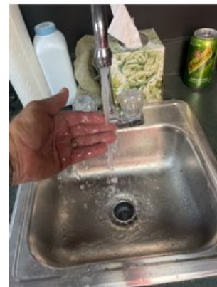
BAR SINK, HOT WATER ONLY, RIGHT SIDE NO FLOW
