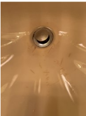
SURFACE SCRATCHING SECOND FLOOR BACK BATHROOM SINK
