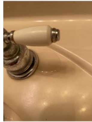
SECOND FLOOR BACK BATHROOM SINK RIGHT SIDE VALVE LEAKS
