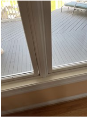
BACK FAMILY ROOM WINDOW GAPPED DOES NOT SEAL
