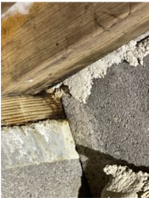
CHIMNEY FRAMING MOISTURE INFILTRATION
