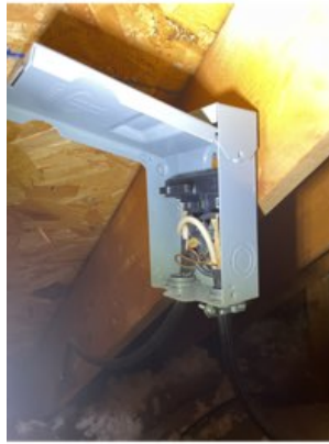
ATTIC HVAC DISCONNECT MISSING COVER
