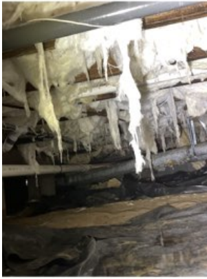
STREAMING INSULATION, SATURATED
