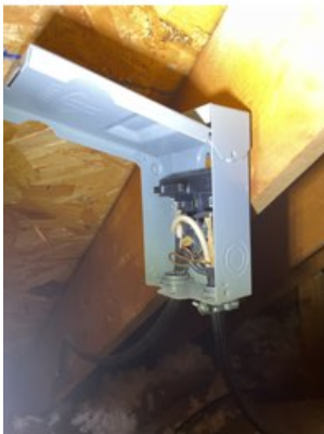
ATTIC HVAC DISCONNECT MISSING COVER
