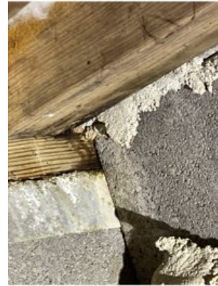
CHIMNEY FRAMING MOISTURE INFILTRATION
