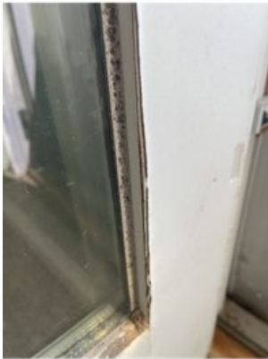
SECOND FLOOR OFFICE DOOR DELAMINATION
