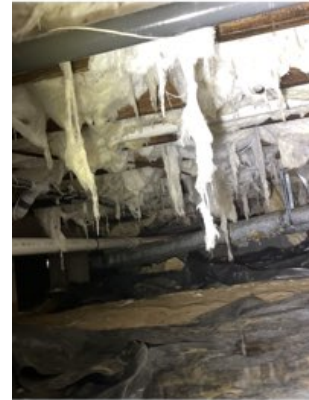
STREAMING INSULATION, SATURATED
