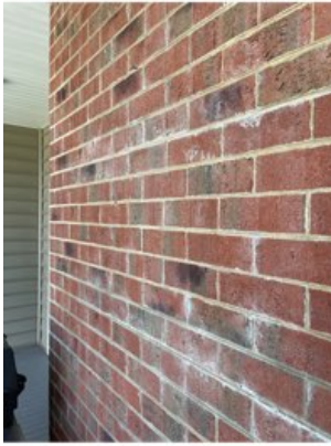
CHIMNEY EFFLORVESENCE
