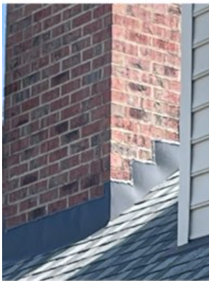
Roof penetrations and flashing
