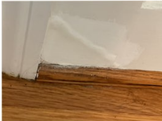
FRONT DOOR, MOISTURE PENETRATION, NOT ACCESSIBLE FROM CRAWL DUE TO WET CONDITIONS
